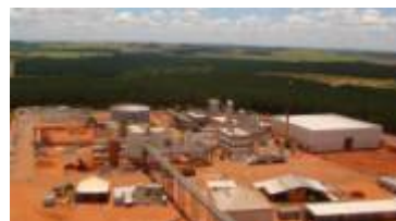
DRI – Resin Plant
