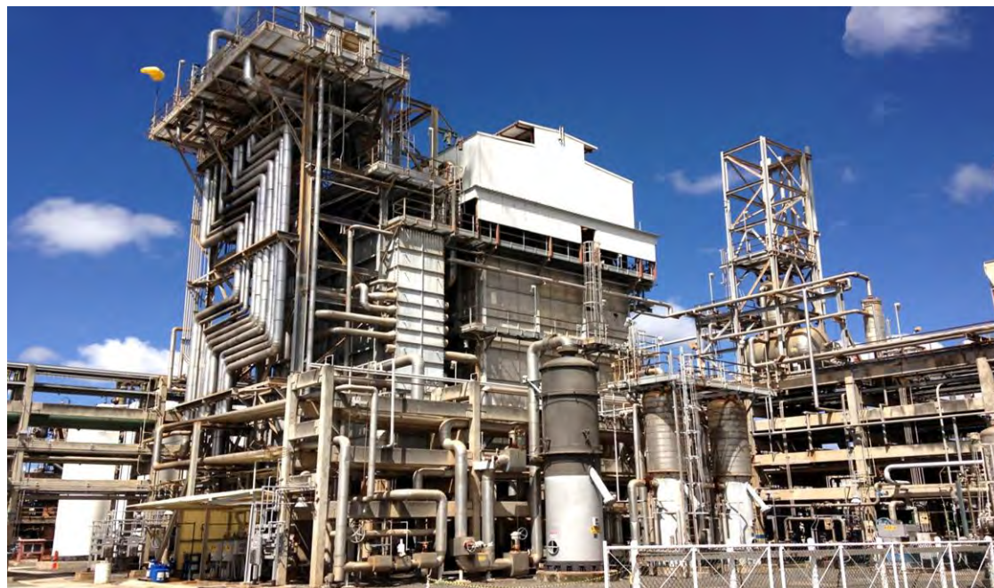
View of the Elekeiroz Industrial Gas Plant
